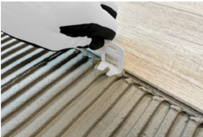
disposable clips installation
