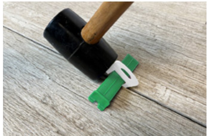
wedges and clips removal
