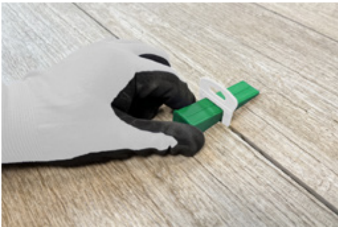
levelling wedges insertion
